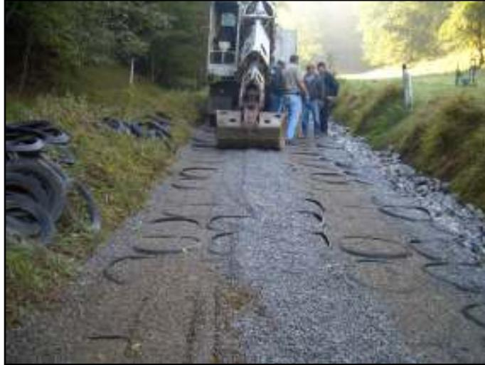
Figure 4 Mechanical Concrete<sup>®</sup> Base
